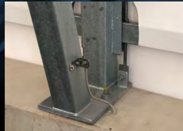
Anchoring on concrete
