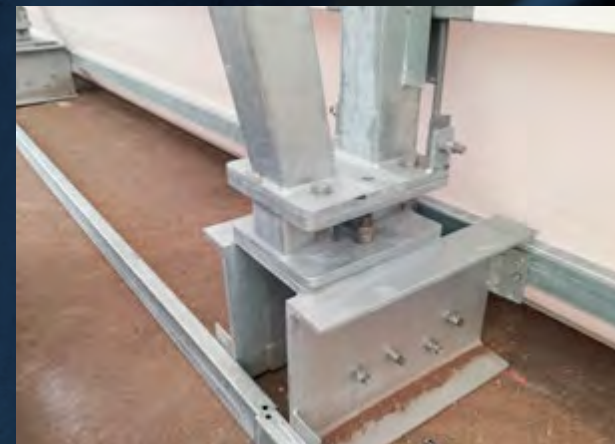
Anchoring on Lürä partition walls
