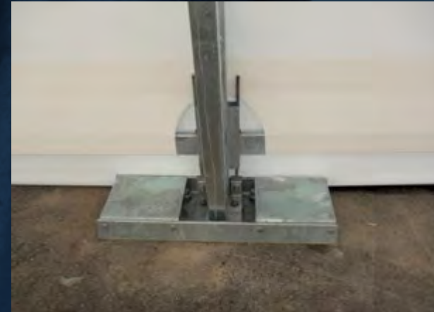
Anchoring on asphalt (injection anchor)
