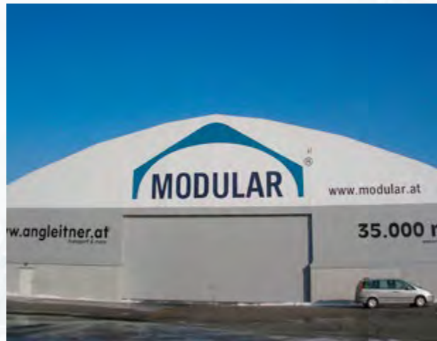
Swing gates and personnel door
