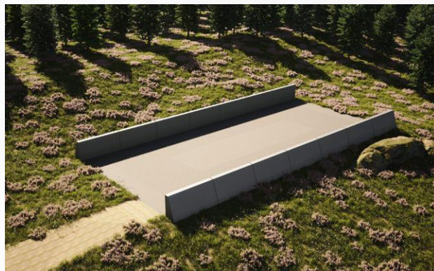
3. Filling of the walls with sand, water, or bulk material.
